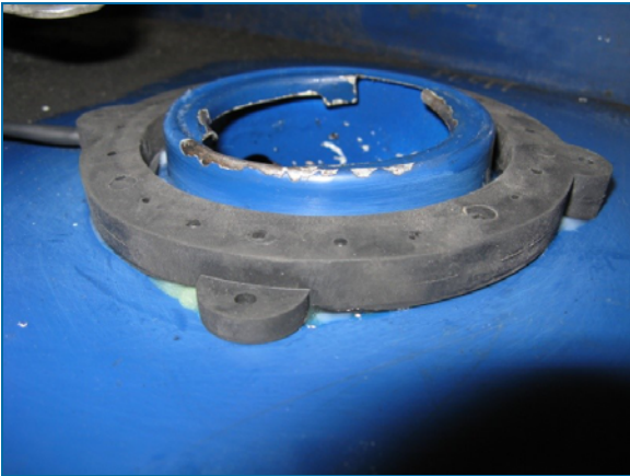
Figure 3-6 Collar Tag Installed on Inlet
