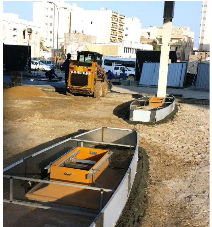
Fibrelite EL-G-E500 dispenser sumps ready for concreting
