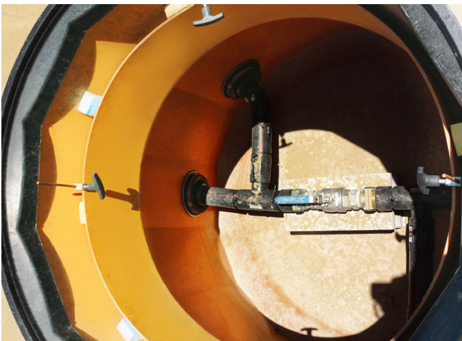
Vacuum testable Fibrelite pipe sealkits form watertight seal
