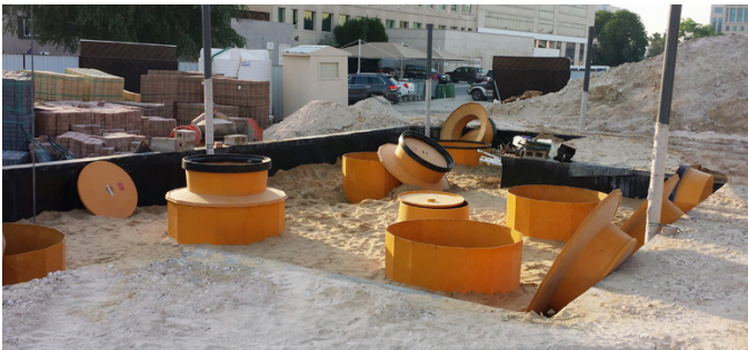
Fibrelite S14-390 tank sumps under installation
